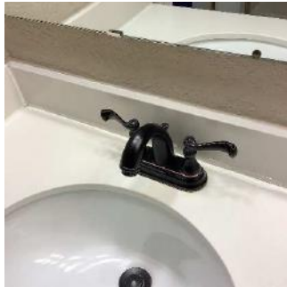
Sink / Faucet (1/4) 05/24/2021 12:06 PM
