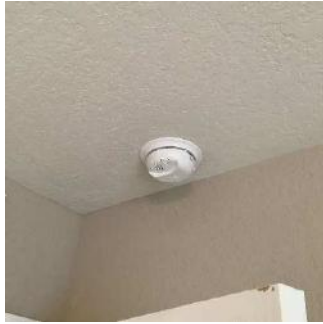
Smoke Alarm 05/24/2021 12:30 PM
