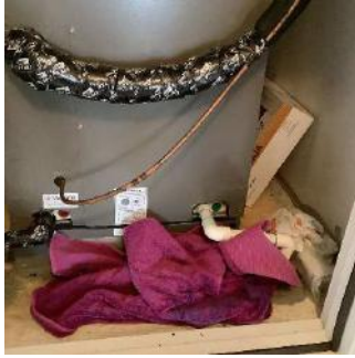
HVAC Return / Filter (Location and Size) (4/4) 05/24/2021 12:29 PM
