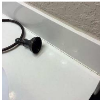
Sink / Faucet (5/5) 05/24/2021 12:35 PM
