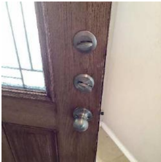
Keyless Lock & Re-keyable Deadbolt Installed (2/2) 05/24/2021 11:45 AM
