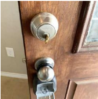
Keyless Lock & Re-keyable Deadbolt Installed (1/2) 05/24/2021 11:45 AM
