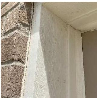
Garage Door Exterior (2/4) 05/24/2021 11:32 AM
