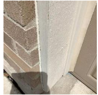
Garage Door Exterior (1/4) 05/24/2021 11:32 AM
