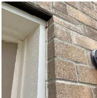
Garage Door Exterior (3/4) 05/24/2021 11:32 AM
