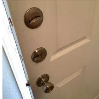
Keyless Lock & Re-keyable Deadbolt Installed (2/2) 05/24/2021 12:10 PM
