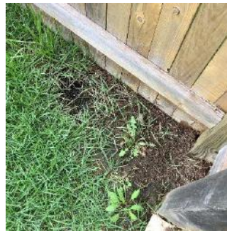
Signs of Erosion/Drainage (1/2) 05/24/2021 11:33 AM
