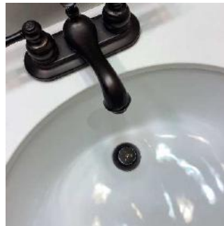
Sink / Faucet (2/5) 05/24/2021 12:34 PM
