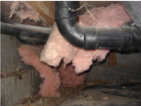
Insulation batts under the floor
