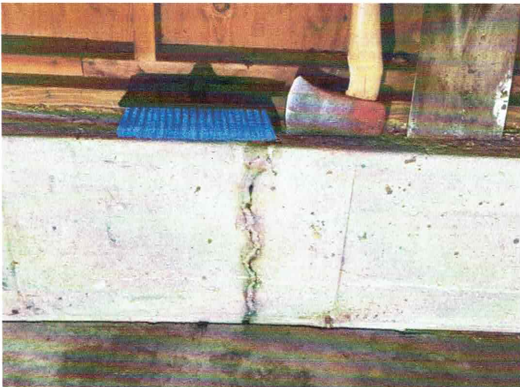
View of rear wall of garage.
