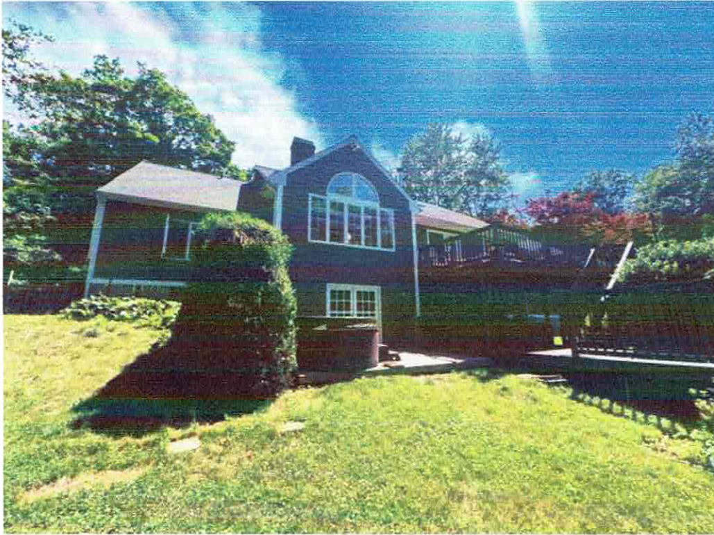
View of rear side of house.
