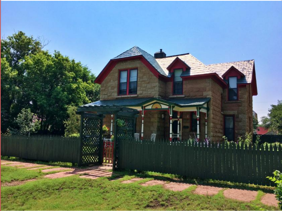
717 Jackson St, above. Built 1890-5. "The porch columns represent yet another design variation in the seemingly infinite array of folk Victorian spindle-work common throughout Las Vegas."
