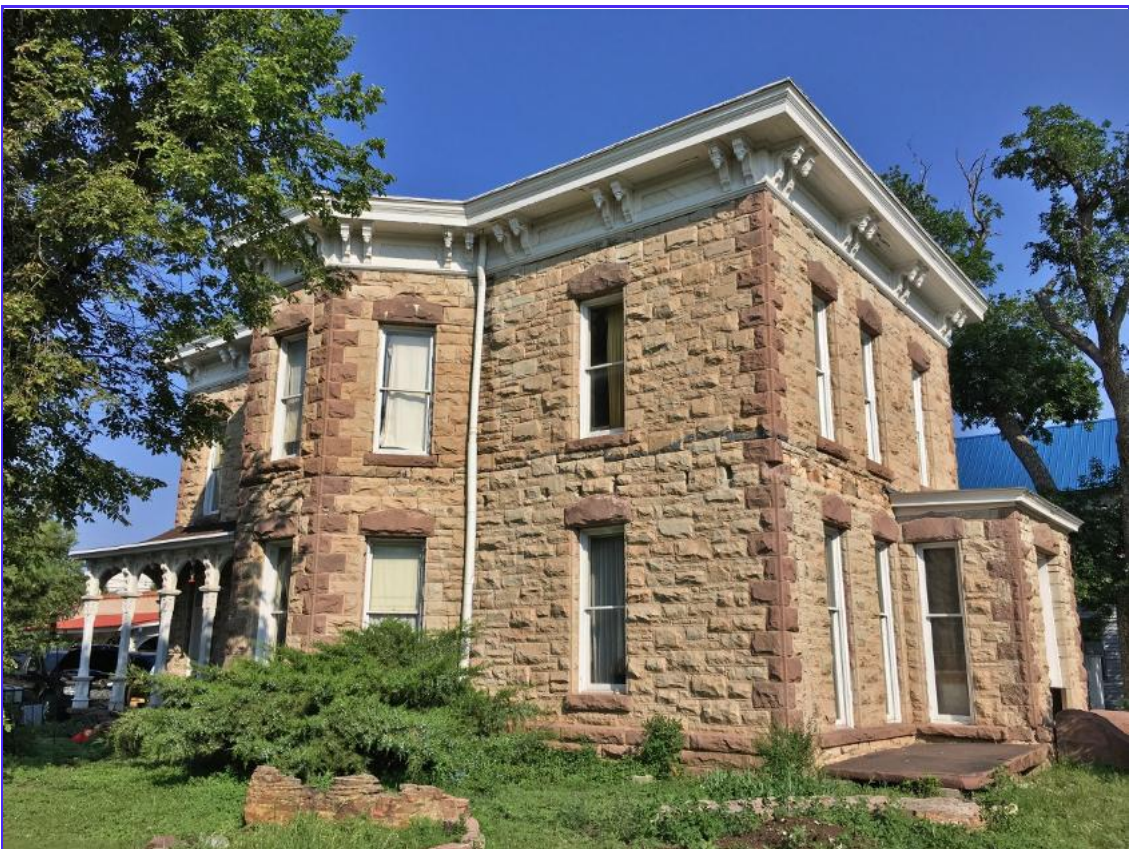
Lutz-Bacharach House 1003 5th St. Built 1884. "This is one of Las Vegas' most imposing
