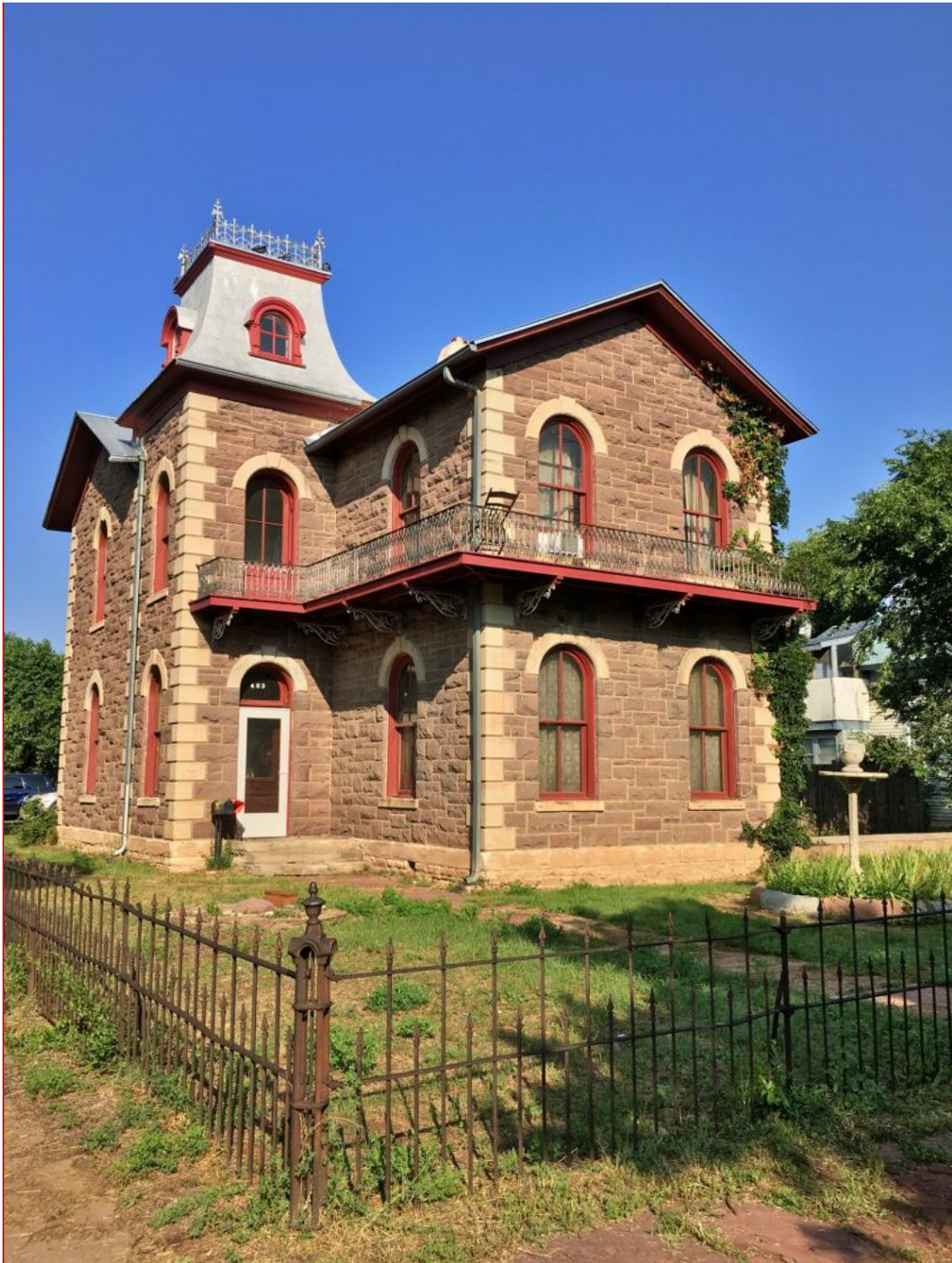
403 8th St. Built 1883. "One of New Mexico's finest Italianate Villas: round-arch window moulding stones contract handsomely with precision-cut brownstone walls; a square corner with mansard roof."
